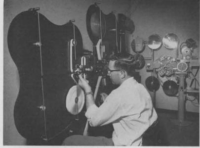
**OPTICAL REDUCTION** printer of the Motion Picture Division 4765 is operated by Gerald Cobb. The machine reduces 35mm film to 16mm. In the background is a double sound-head black and white printer which simultaneously reproduces sound track and film.
